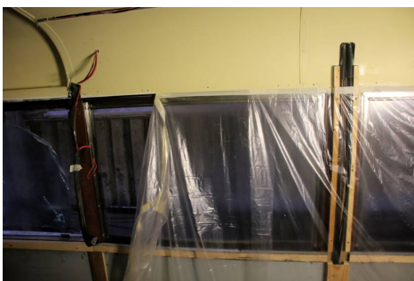
New wiring has been installed. [D G Chick]
