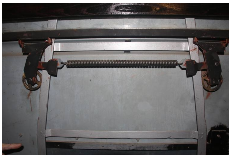
The restoration work is being carried out to a very high standard. This shows the mechanism for the full-drop windows which were necessary in the heat of South Africa. [D G Chick]
